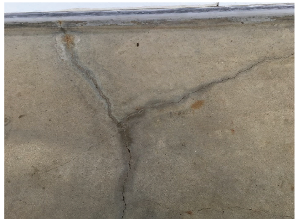
Figure 3 Floor cracks effectively harbour pests and pathogens during cookout. Image: Warwick Gill
